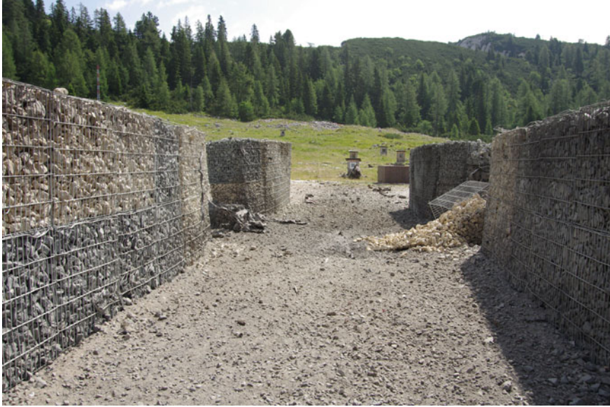
Fig. 7.9 Gateway as shown in Fig. 7.8 after the explosive event. The gabions are seriously damaged near the original location of the car bomb. Some of the gabions at the right hand side tumbled back in the direction of the hazard source, because behind them a further test vehicle was located for damage assessment. The crater is comparatively small because of the rocky ground. In the middle of the picture, fragments of the car and protective structures for the filming and measuring equipment are visible. For instance, a massive fragment lies just straight ahead. Also the radial segment markings for locating the fragments are visible, see the thin white lines that originate from the explosive source location (Technical test center WTD 52 2013)
